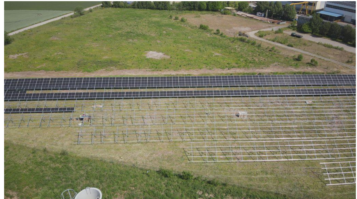
photovoltaic farm under construction
